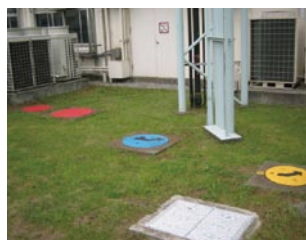
Color-coded manholes
