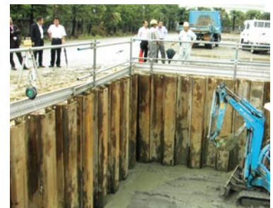
Contaminated soil removal by excavation
