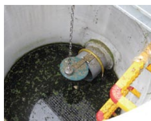
Newly installed emergency shutoff valve
